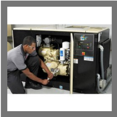
Air Compressor Repair Services
